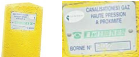
(Borne qui matérialise le passage de la conduite)
